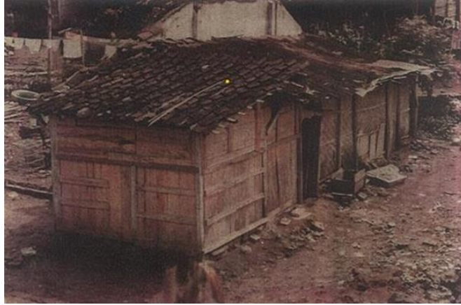
Figure 3. The New House Building of Pawirorejo besides the Original House Building Remnants
