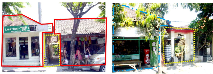
Figure 5. The traditional wall and gate have been demolished
